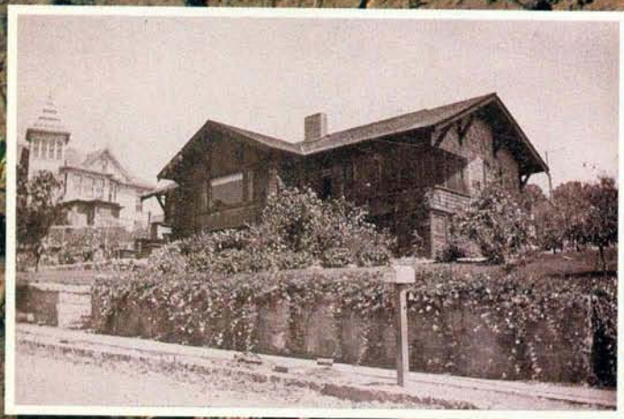
ABOVE: Contractor Steve Crawford reframed almost all of Jan Winford's house, but he's putting back the signature elements of the Arts and Crafts style—low-pitched gable roof, brackets, and wide overhangs. LEFT: Before its reconstruction, the shape of Jan's bungalow hadn't changed much since this picture was taken in 1914.
