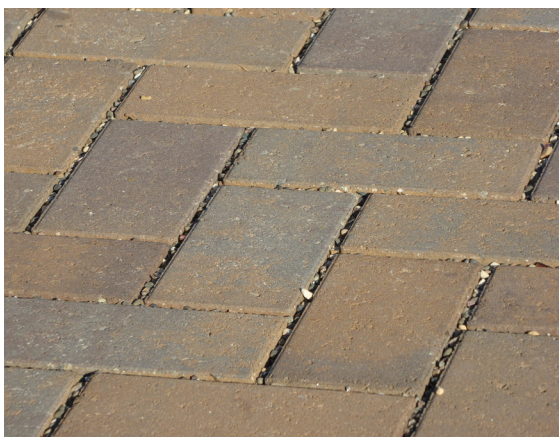
Special pavers let water percolate into the soil. Gaps between flagstone slabs keep oaks happy.
