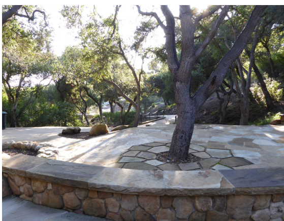
Special pavers let water percolate into the soil. Gaps between flagstone slabs keep oaks happy.
